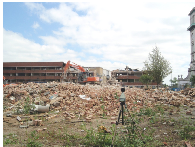
Monitoring noise during demolition
