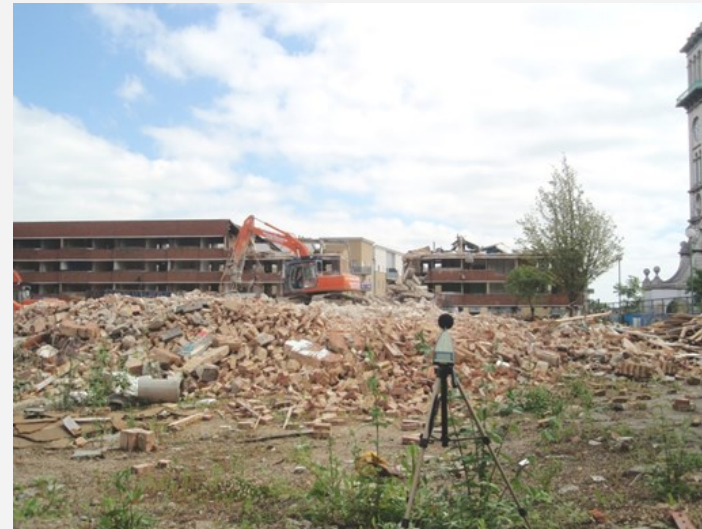
Monitoring noise during demolition
