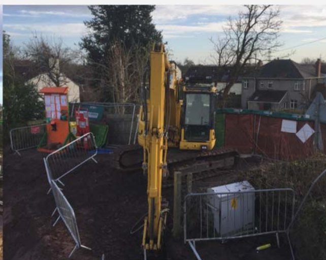
Bridge replacement works underway with housing nearby
